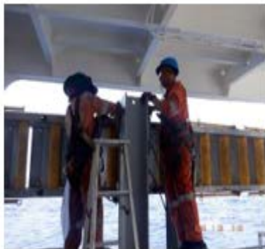
Working on port side
